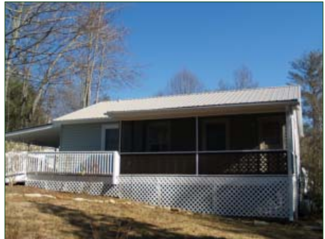
Front from street
