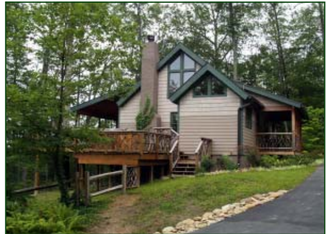
Paved streets and driveway
